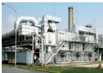
Kyoto Works VOC disposal facilities (heat-storage type deodorizing furnace)
