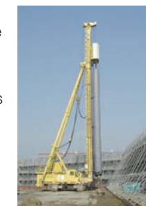
Installation of submerged permeable reactive walls
