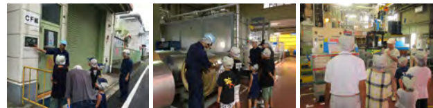
Plant observation tour at the Kobuchizawa Works
