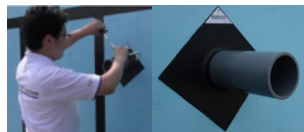
Example of construction of air-tight materials
