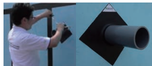
Example of construction of air-tight materials
